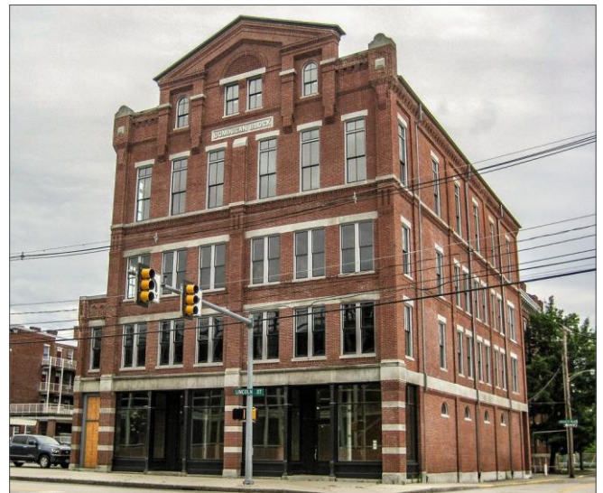
The Dominican Block was restored with contextually appropriate windows and masonry. Photo by Lyme Properties.
