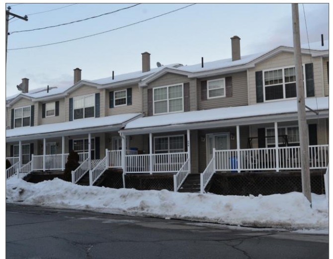
Roofs shall be designed to prevent falling ice and snow onto entrances and walkways. Photo by Craig Saddlemire
