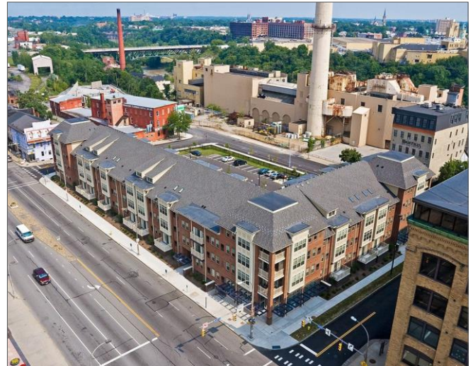
Parking areas shall be located within the interior of the site to minimize visibility from public streets and parks.
