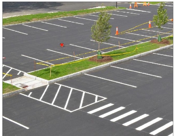
Pedestrian and vehicular crossings shall be clearly marked, using signage, curbs, pavement striping and/or special paving materials. Photo by MBTA
