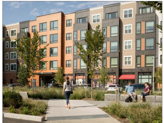
The front setbacks of multi-use buildings can use landscaping with a mix of green and hard surfaces to create a sense of place.
