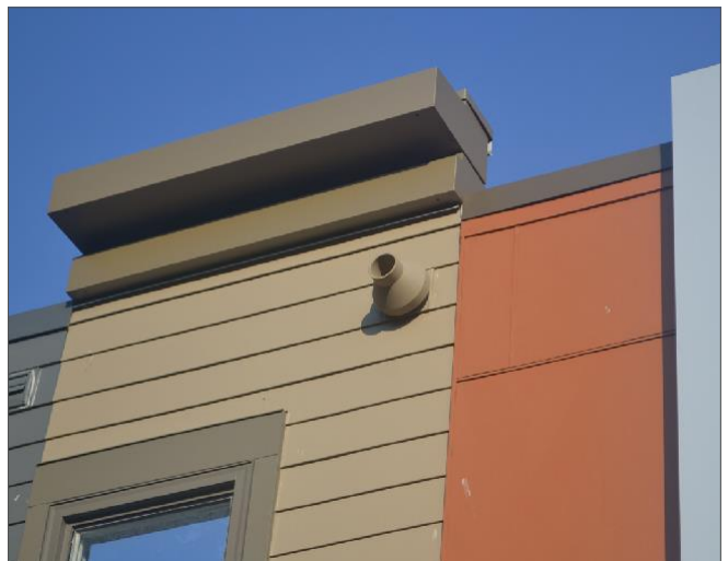
Exhaust vents and other mechanical attachments, where present, should match the facade.
