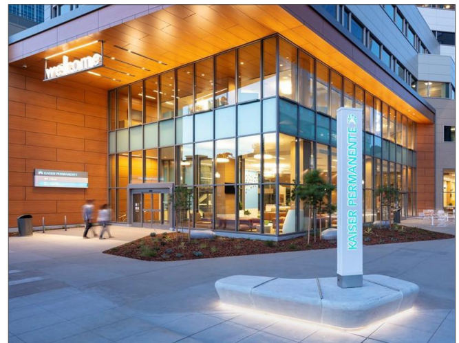
Commercial and institutional front setbacks should emphasize public entrances with expanded sidewalks. Trees and plantings are encouraged.
