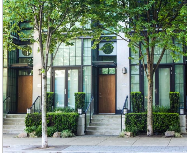
Ground story dwelling units shall be elevated at least 21 inches above the grade of any adjacent sidewalk.
