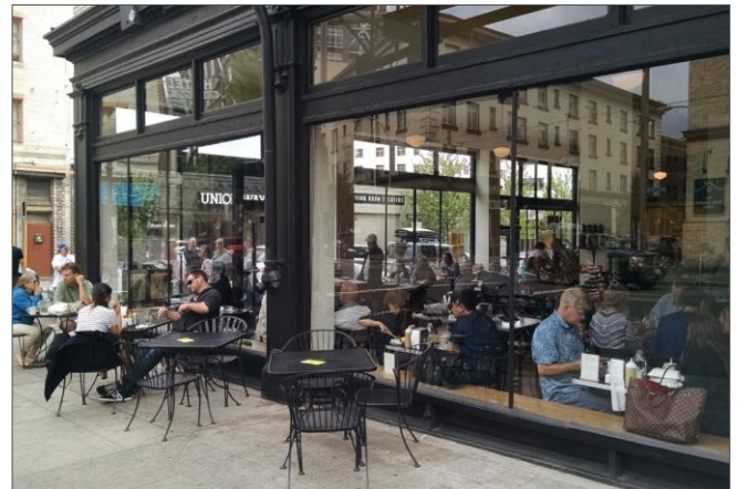
First floor commercial clear glass example. The actively used area should have a depth of at least 20 feet, or the depth of the building if less.
